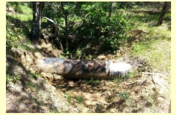
This photo shows an exposed section of the 90-year-old “Gordon Line” just south of Lake Curry. The Gordon Line once transported large quantities of water from Lake Curry to the City of Vallejo. Today, water is reverse fed up the Gordon Line to serve a few end users in Gordon Valley.
